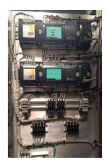
The BFM-II is ideally designed to upgrade existing substations with electro-mechanical relays to provide real-time information and management lacking in these highly reliable devices.
